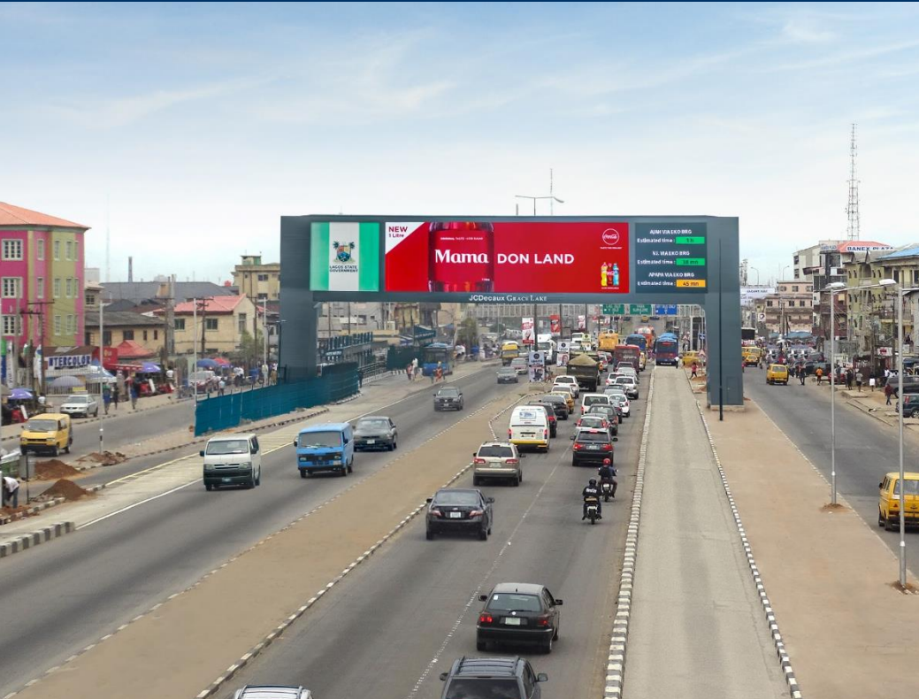
92sqm LED gantry providing real-time traffic info, Lagos, Nigeria
